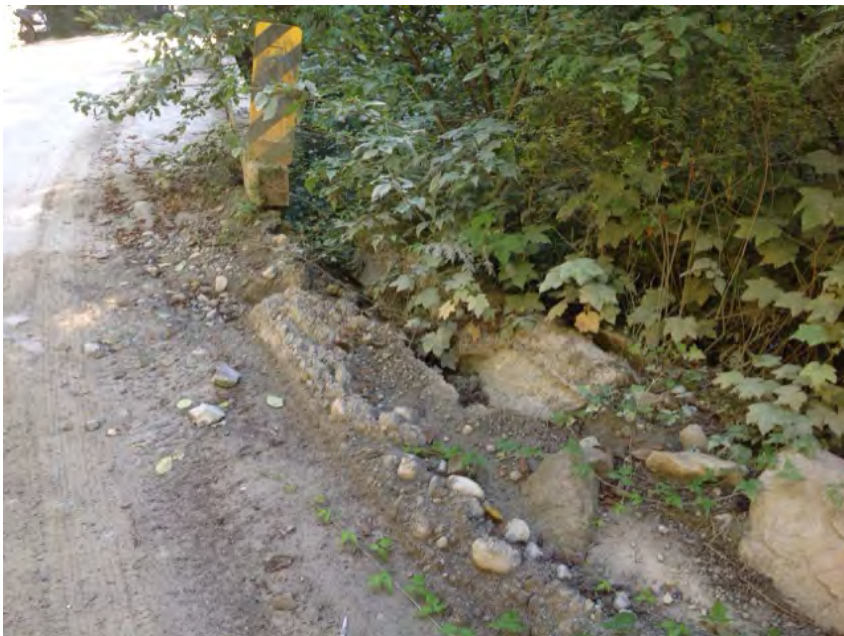
right bank downstream no post
