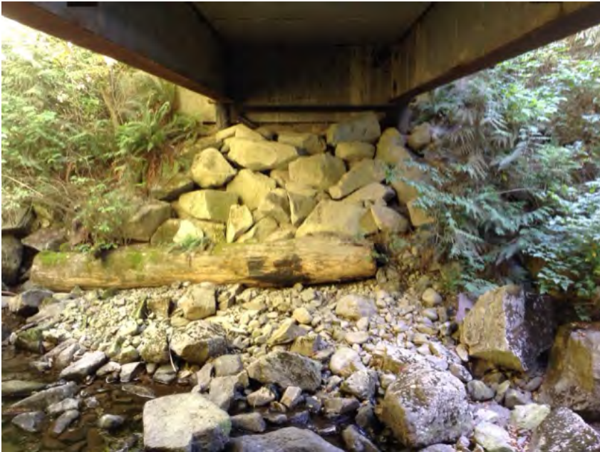
Left Bank Abutment when facing downstream
